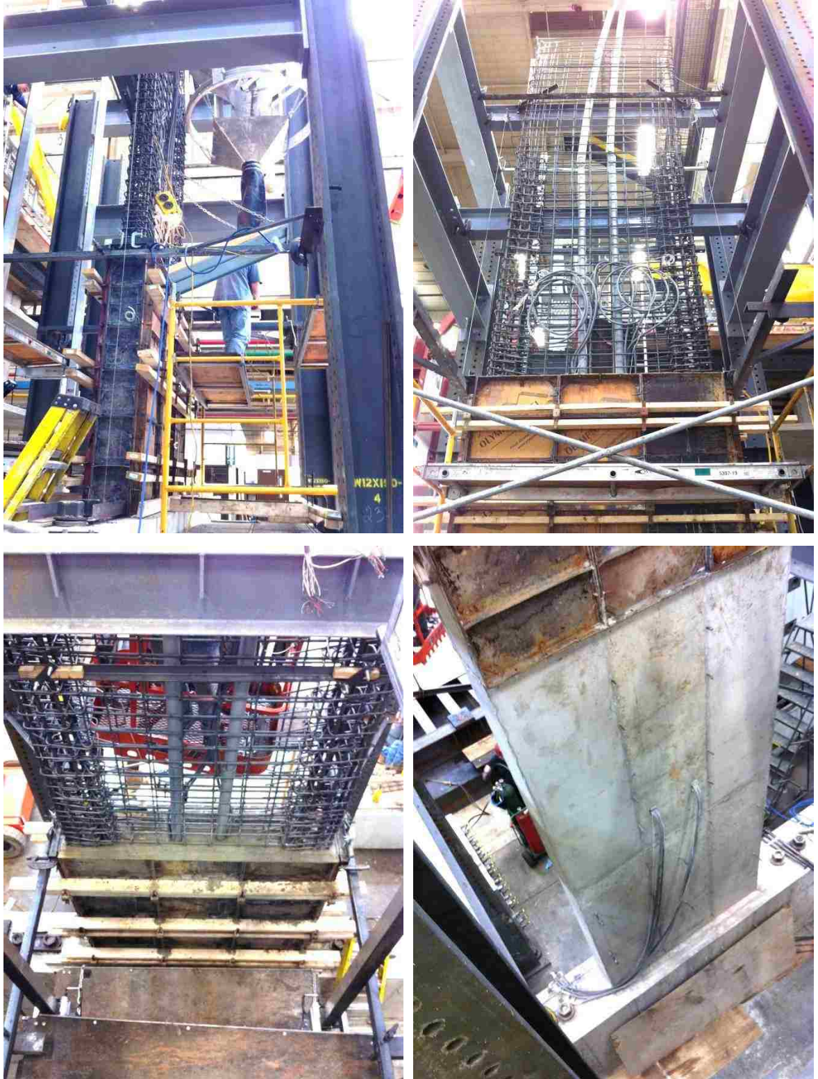
Figure 3-24 Additional construction photographs
