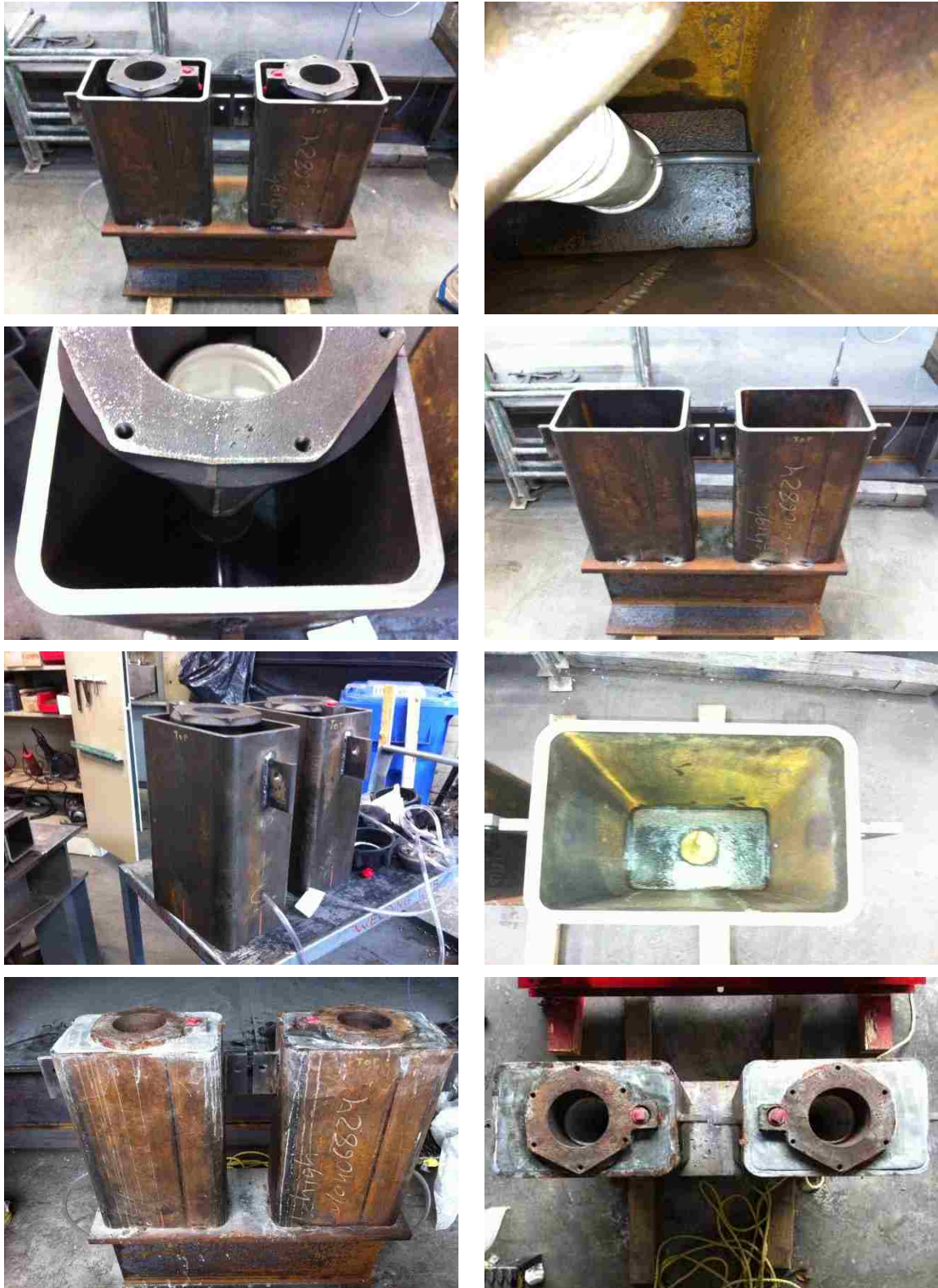
Figure 3-12 Construction photographs of the top anchor head encasement
